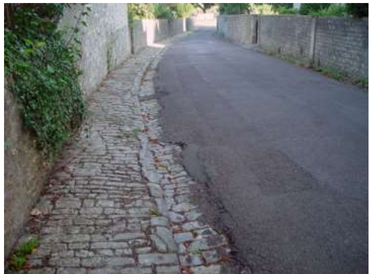
Varieties of laying-patterns found in pitched walkways throughout the district, at Chew Magna (left) and Newton St.Loe (right)
