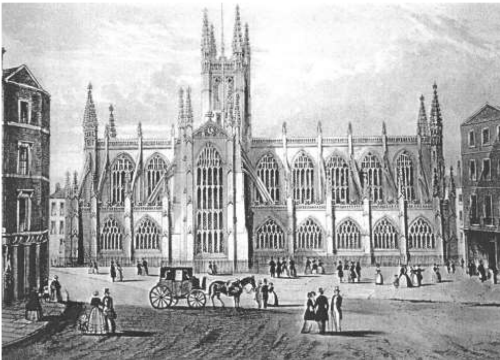
Below: The lower end of the High Street c.1850, by J.Newman. The flat pedimented face and part of the rounded SW corner of Nos.1 and 2 High Street is visible on the far left. From Illustrations of Bath and Vicinity .
